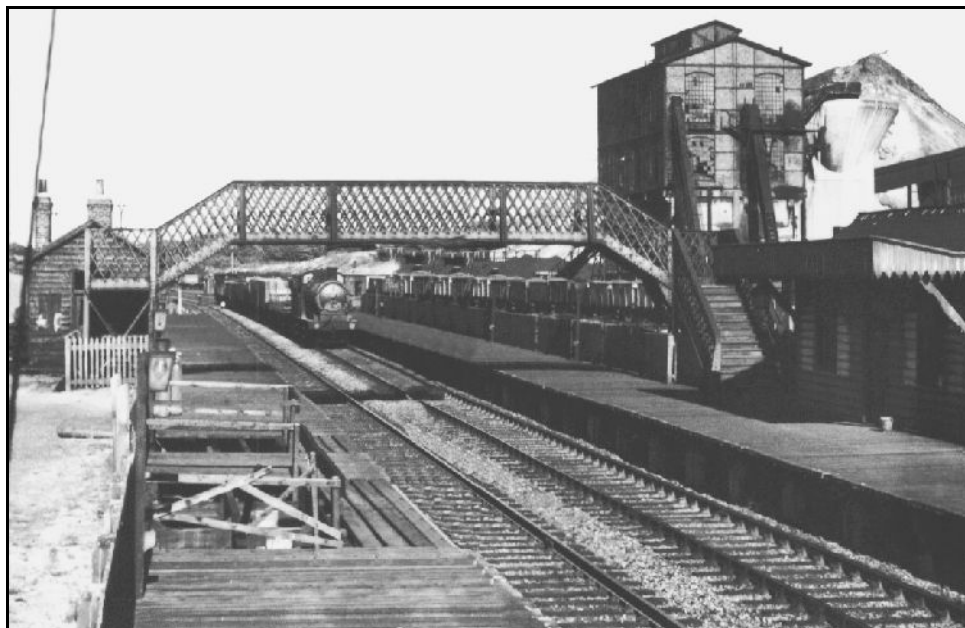
BR class J11 0-6-0 no.64451 passes through Waleswood station with a westbound goods on 3 rd July 1955. Waleswood colliery is on the right. photo: H.B.Priestley/J.Howard Turner collection
